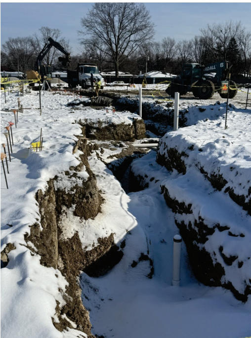
Underground Plumbing Main Corridor
